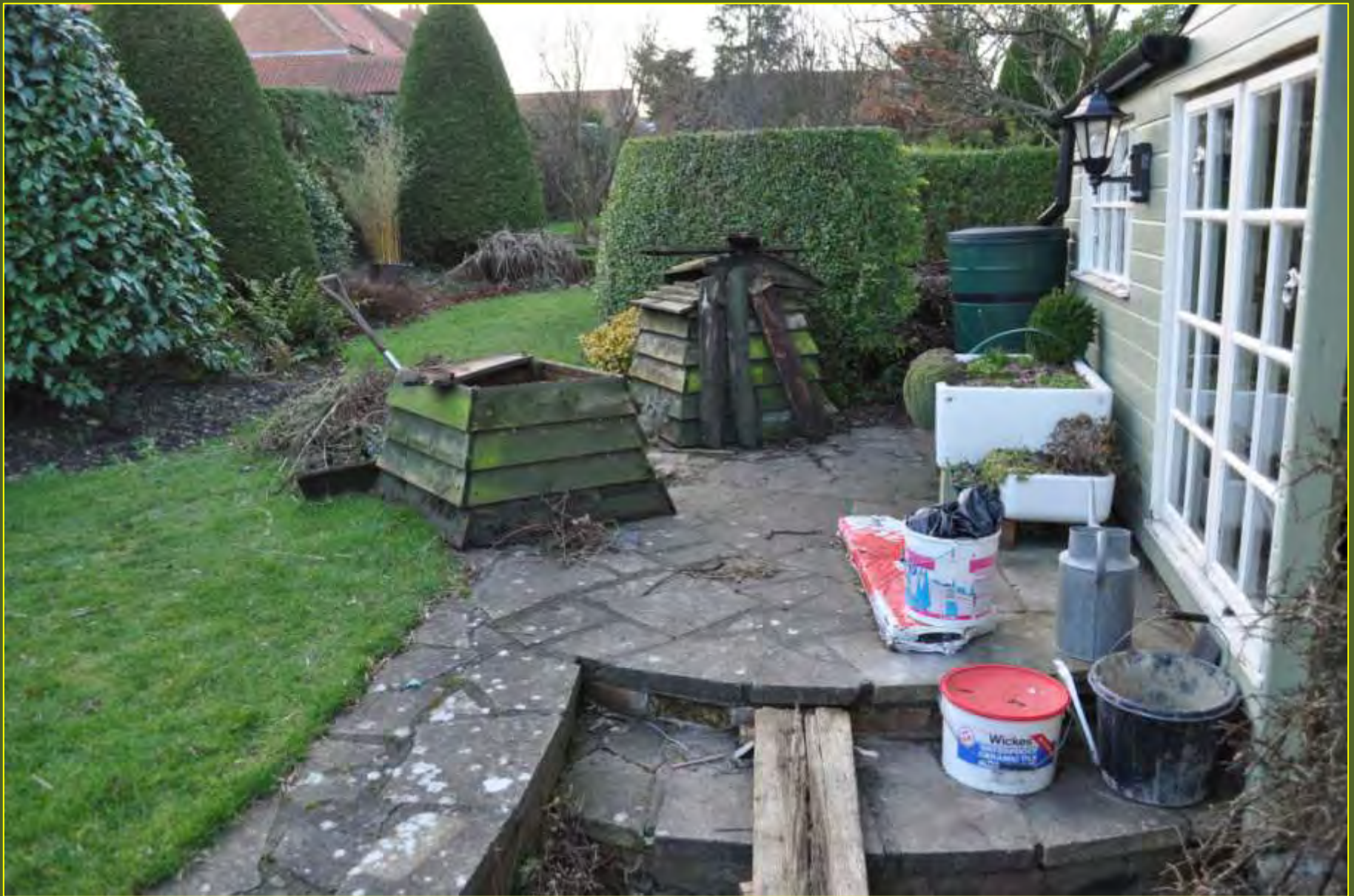
Hive bins in need of repair. Rotting despite being tanalised
